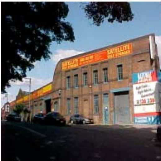
Photo: Federation period warehouse on Booth Street.
