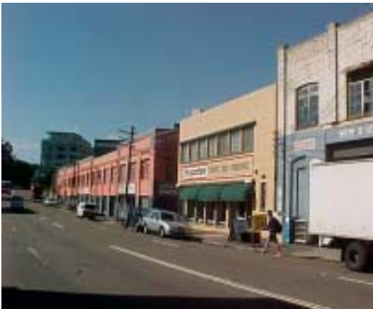
Photo: Industrial development built to street alignment along Pymont Bridge Road.
