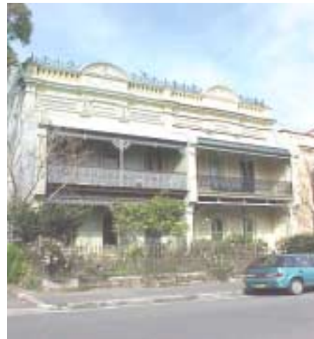
Photo: Row of Victorian Italianate terraces located on higher slopes of the Neighbourhood.
